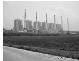
Power Plant in Korea
